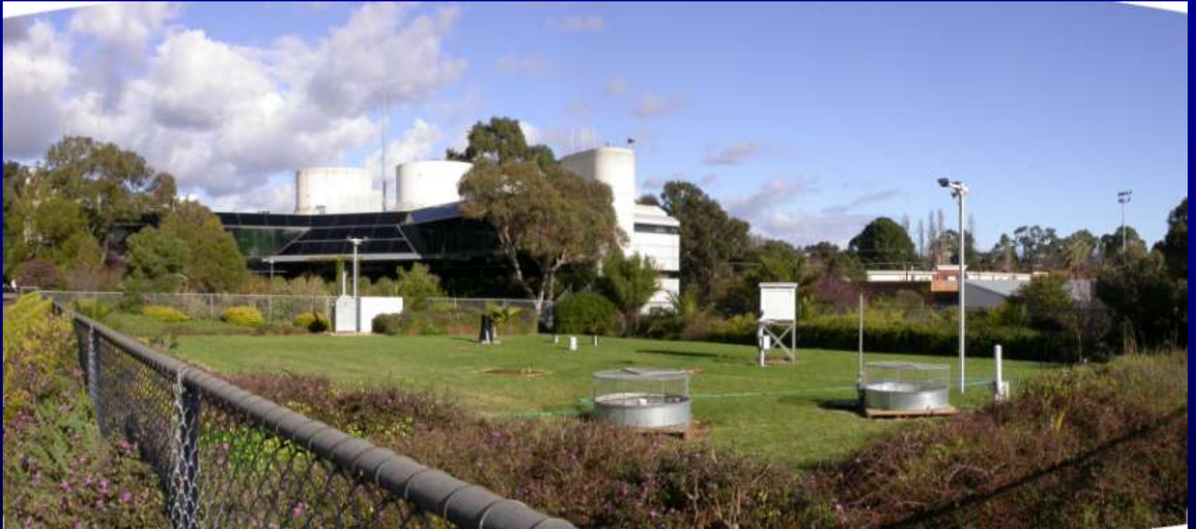
The BoM weather station, Kent Town
