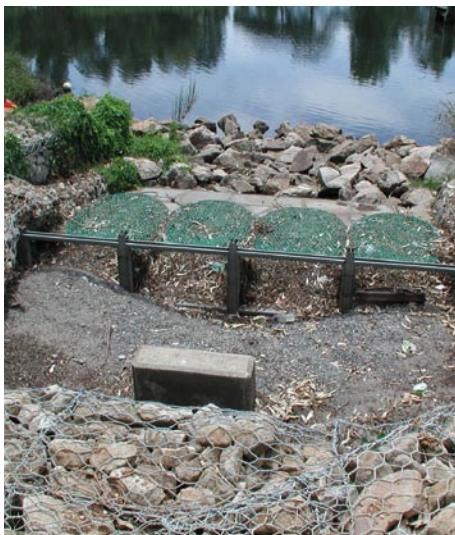
Sediment and vegetation debris collected in trash rack after flow (photo: Allin Hodson)
